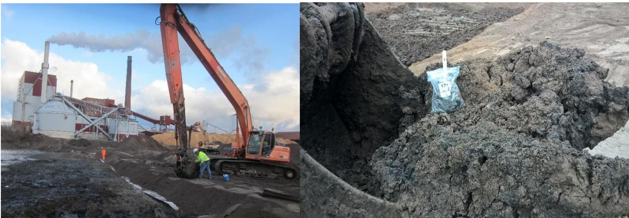
Figure 7. Sampling for technical testing during stabilization works.
