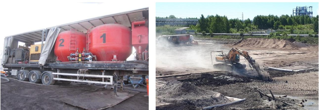
Figure 12. Dry binders were mixed on site by blowing them in different tanks several times before the mass stabilization. Two different binder mixtures (e.g. fly ash and cement) can be fed at the same time to the excavator with mass stabilization equipment.
