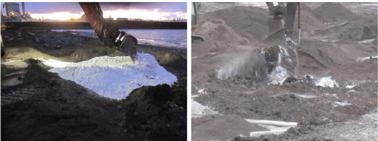
Figure 5. Spreading and premixing of gypsum waste to sediment with excavator.
