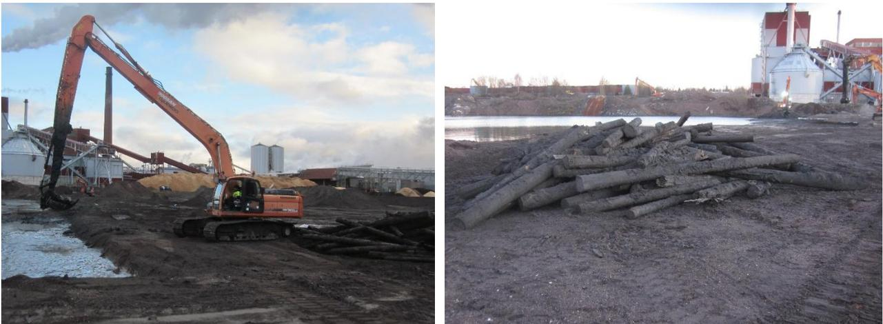
Figure 4. Removal of logs from the basin before mass stabilization carried out by excavator with attached rake head
